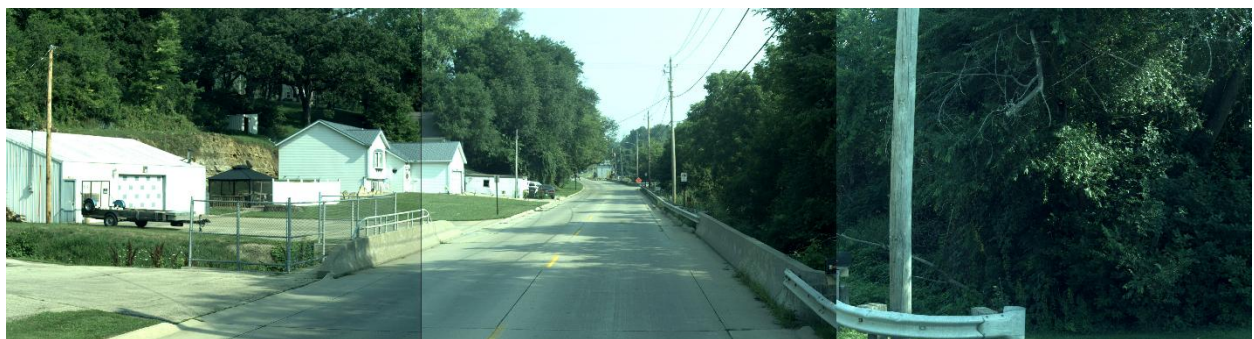
Figure 232: W-Beam Guardrail and Pedestrian Water Crossing along Peru Road (Image Source: Pathweb )
