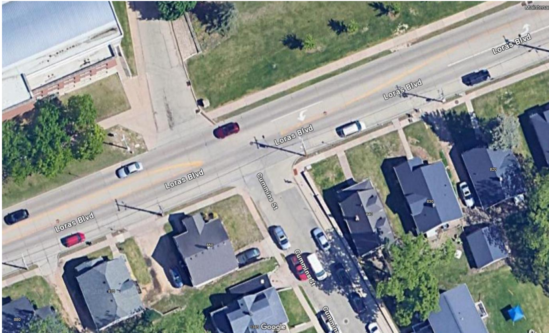
Figure 154: Intersection of Loras Boulevard and Cummins Street
