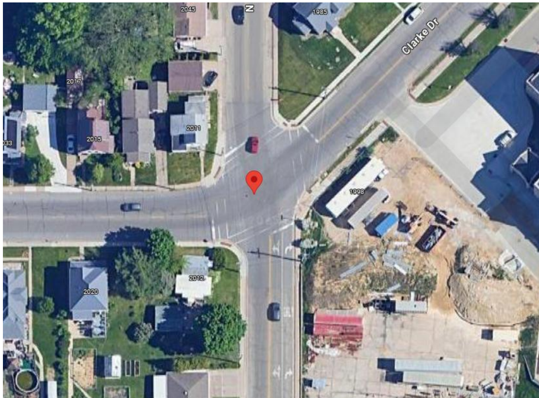
Figure 191: Intersection of Clarke Drive and Grandview Avenue
